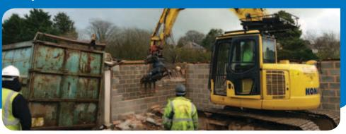
The site compound is now set up within the car park. Works are progressing well - the garages have been demolished and the rubble is being crushed to reuse on the site.
