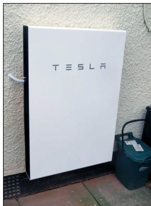
Figure 2 External Tesla Powerwall 2 installation
