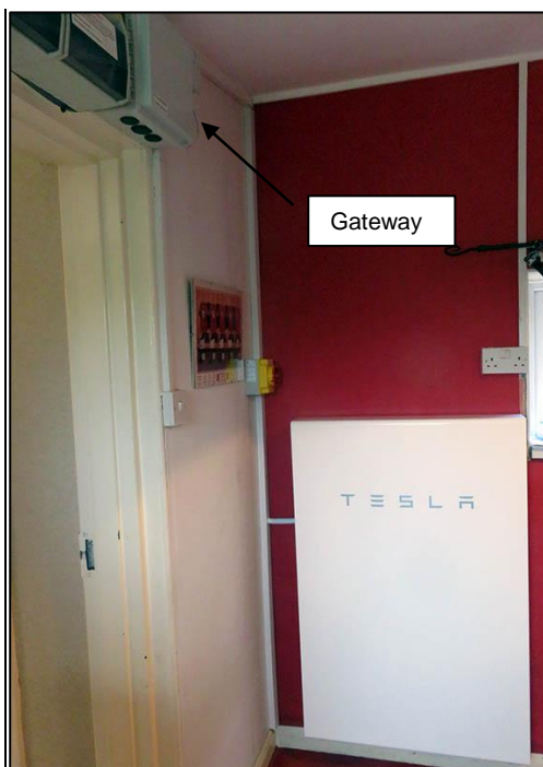
Figure 1 Internal Tesla Powerwall 2 installation
